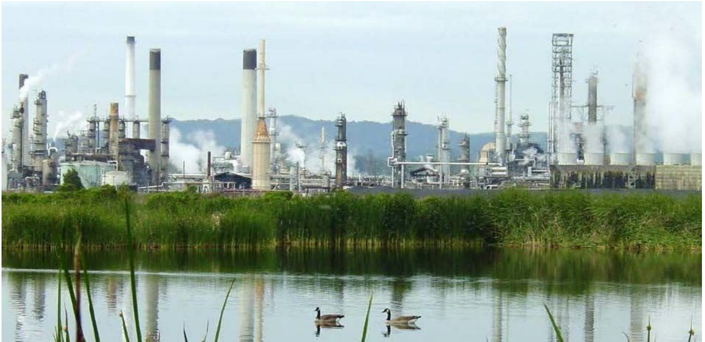
Marathon's refinery in Martinez, CA. Source: Contra Costa County site
